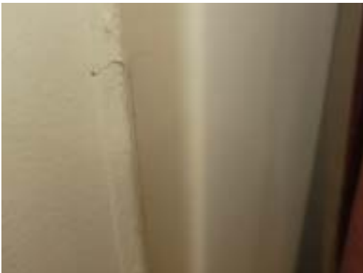
2715-11 Caulk Interior Bathrooms/Sinks/showers
