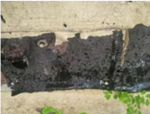
2715-3 House Wrap/Tar Paper Typical Exterior Walls
