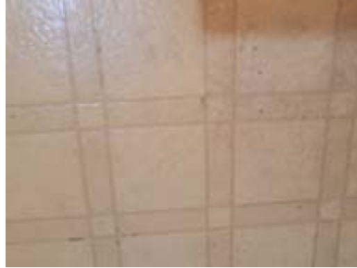
2715-8 Rolled Flooring/Mastic Interior Hall Bathroom
