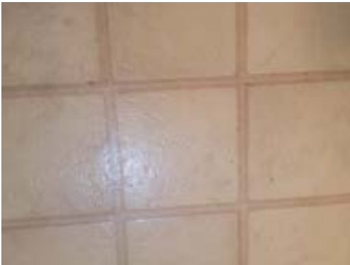
2715-9 Rolled Flooring Interior Master Bathroom
