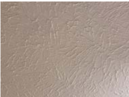
2715-5 Ceiling Texture Typical Interior
