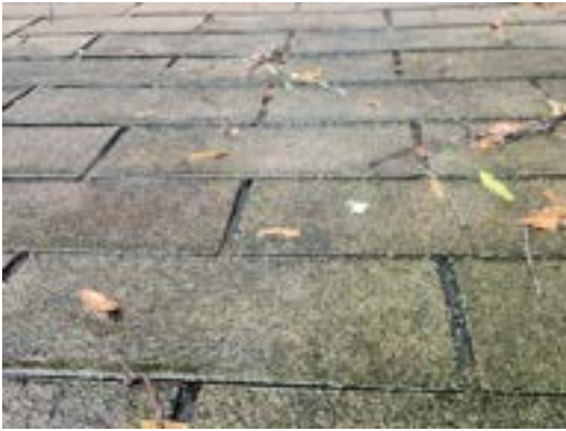
2715-1 Asphalt Shingle/Tar Typical Exterior Roof
