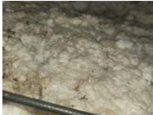
2715-10 Insulation Interior Attic Crawlspace
