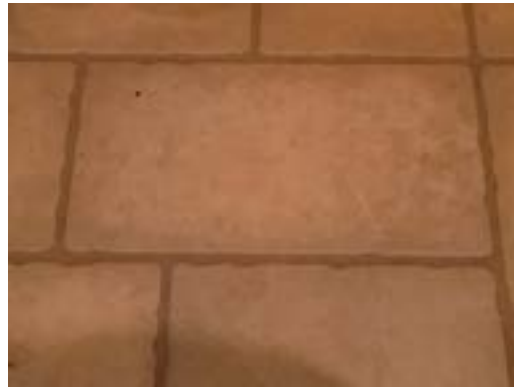
2715-4 Rolled Flooring Interior Kitchen/Front Entry
